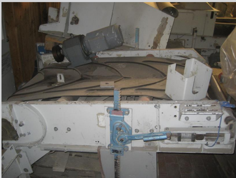
Bag discharge belt conveyor
