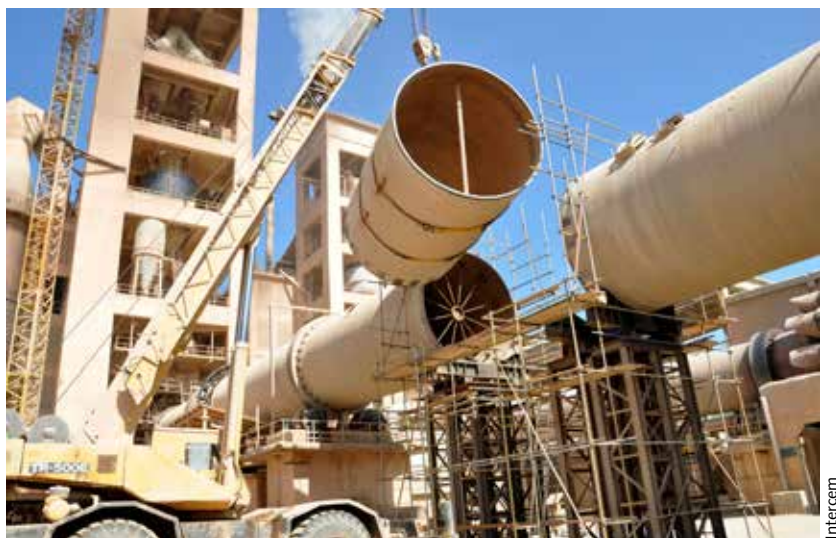
7 Setting up a rotary kiln in Tanzania (TWIGA)
