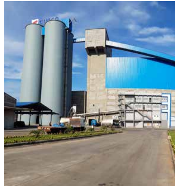
4 2.5 million t/a cement grinding plant with VRM in West Africa
