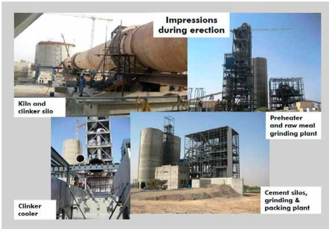
5 PAN Emirates Cement; Phase 2; Layout, design and commissioning of a complete 2400 t/d cement plant with Semi-Turn-Key delivery of core equipment
