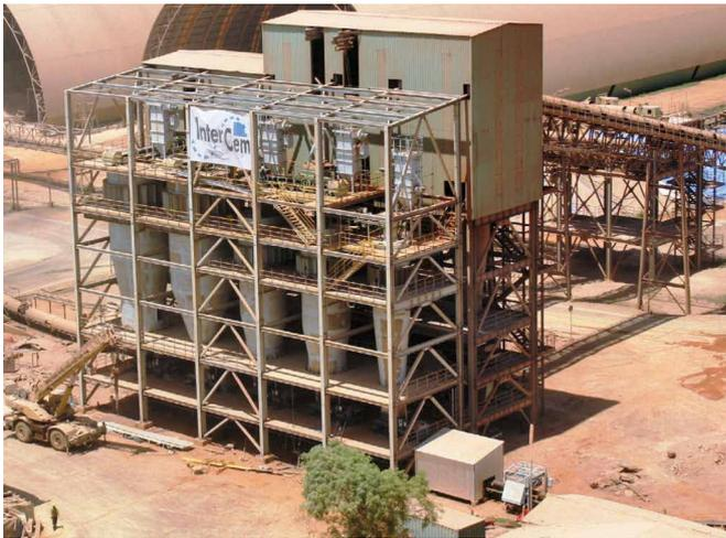
**3** New raw material preparation station for HGL / LGL / Gypsum, red soil and iron ore
